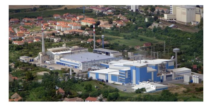
The main part of the facility which serves for the manufacture of glass fibre comprises a glass manufacturing plant measuring  $150 \times 150$  m. The plant includes several separate sections: a transformer station, raw material feeding bins, preparation of raw materials, product processing, recycling, storage area and others.
